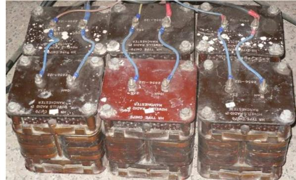
Fig.6 active filter inductor
