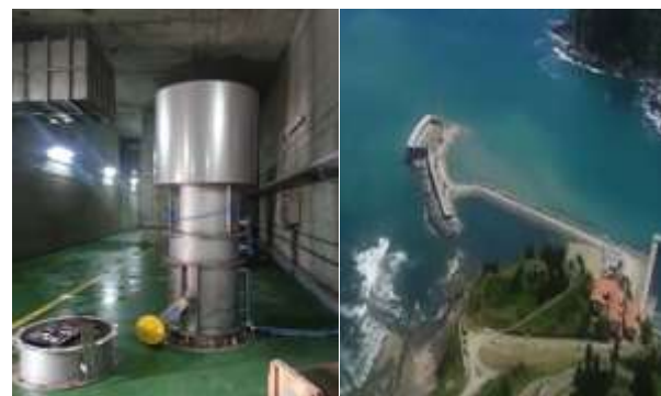
Fig. 1: Turbo-generator modules employed within the Mutriku wave plant
