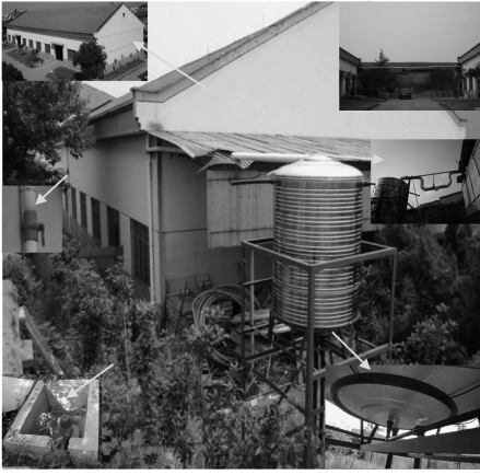
Figure 3: Rainfall harvesting device implemented at Zhejiang province
