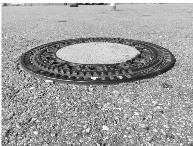
Figure 4: Picture of the overdriven manhole cover to measure the sound pressure level.
