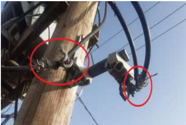
Fig. 10: DT Operating without HRC Fuse
