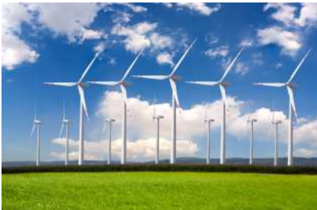
Fig. 4: A wind farm
