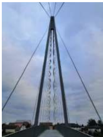
Fig. 4: View of the steel pylon
