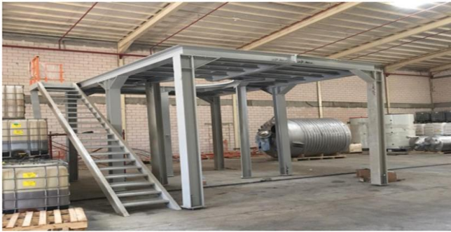
Figure 8: Part of infrastructure inside the factory
