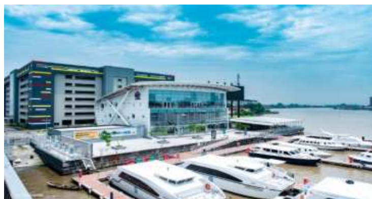
Figure 3: Modern Jetty at Ferry Terminal in the study area Source: Author, 2021
