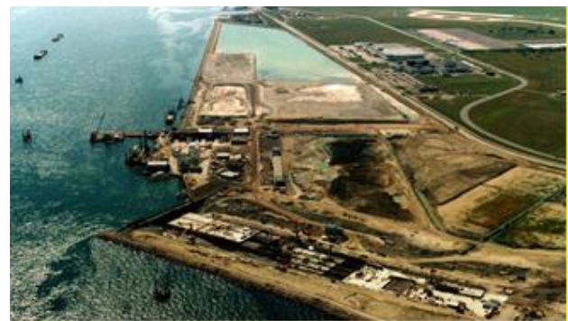
Fig. 6 Tunnel of the Øresund Bridge [22]
