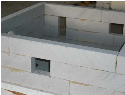
Figure 2: AAC external walls building
