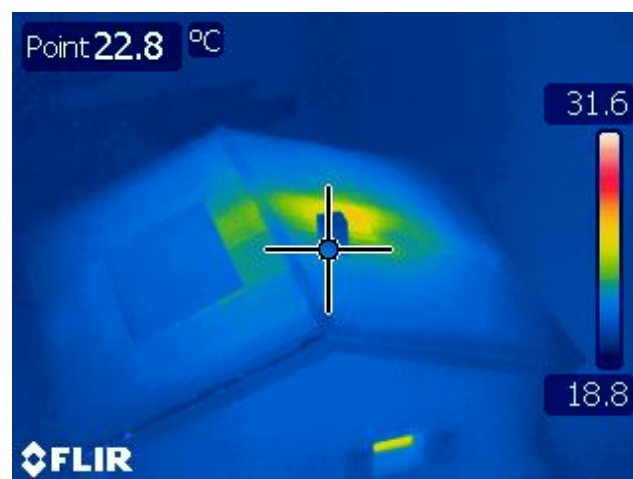
Figure 17: Roof top view with double wall and ceiling insulation
