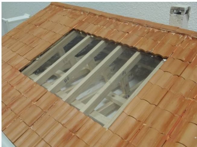
Figure 6: Wood parallel roof truss (pine wood), red tiles, chimney and roof solar panel place
