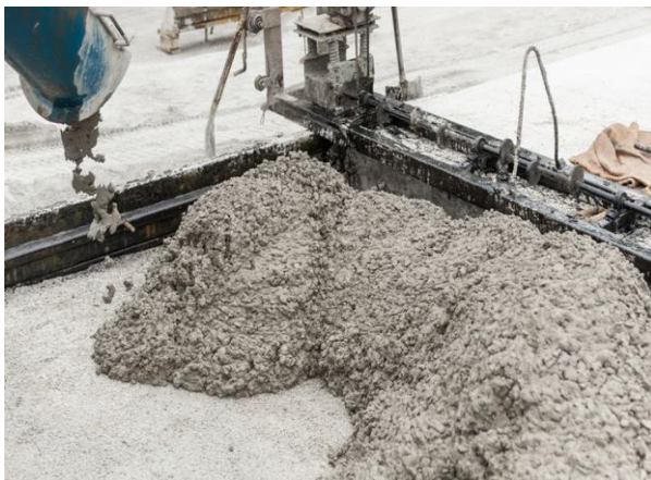
Fig. 7: Placement of fresh concrete during pavement construction.
