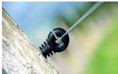
Fig. 5: Ring insulator through which the rope passes, [10]
