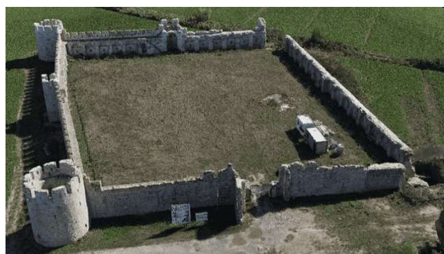
Fig. 7: Point Cloud generated from Terrestrial Laser Scanning
