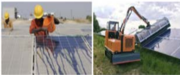
Fig. 3: Traditional and advanced methods of cleaning the solar panels
