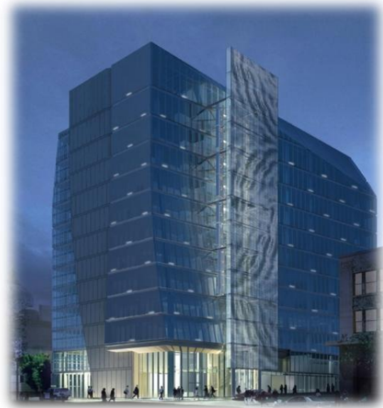
Fig16: The majority of the south facade has fixed shading devices protruding from its high performance glass skin. Automated exterior blinds shade the upper most levels [18].
