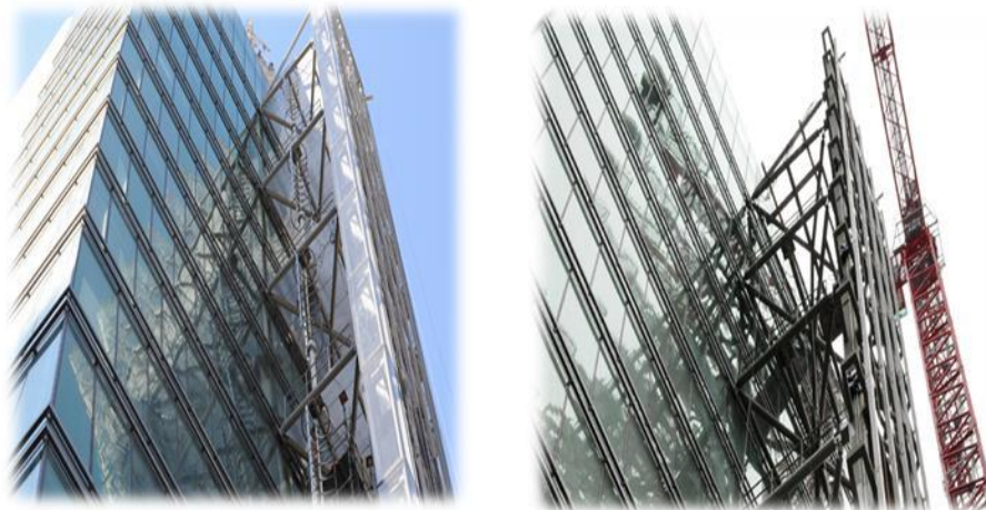
Fig. 19: Completed view of the building's wind turbine helping to create an energy-efficient setting for SFPUC staff.
