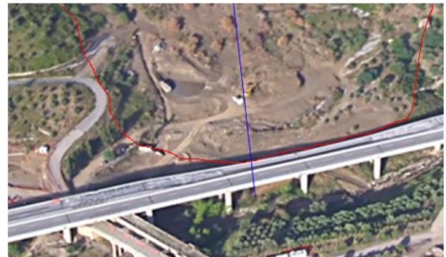
Figure 13 - Orthophoto returned by UAV with delimitation of the landslide area (in magenta), representation of the contour lines (in red) and indication of the section considered (in blue) for the evaluation of displacements. Example applied on Himera viaduct.
