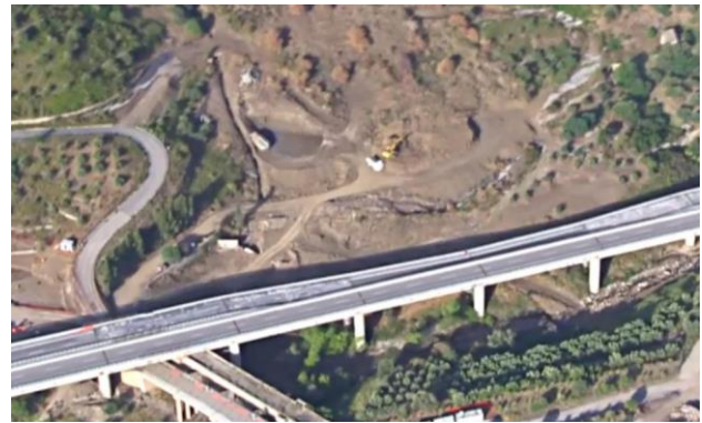
Figure 3 - Landslide close to the HIMERA viaduct.
