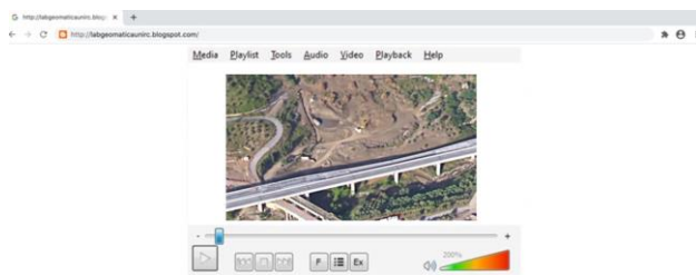
Figure 15 - Frame from the video Himera viaduct example.
