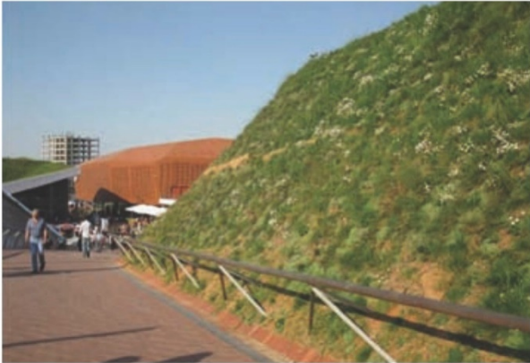
Fig. 5. A vegetated steep slope, at Meydan Shopping Mall, Istanbul, Turkey. Design by Foreign Office Architects (Esbanh, 2011) [12]
