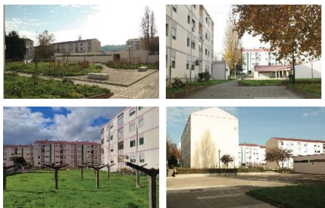
Fig. 2 – Existing situation: (top-left) north entrance; (top-right) view to the commercial 1 floor building; (bottom-left) clotheslines; (bottom-right) southwest entrance.
