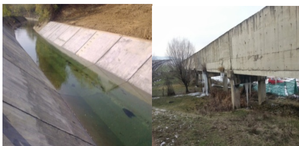
Fig. 6&7, The open canal and aqueducts
