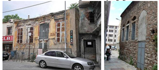
Fig. 15 a) Beit Hillel Synagogue before restoration [10] b) Portekiz Synagogue
