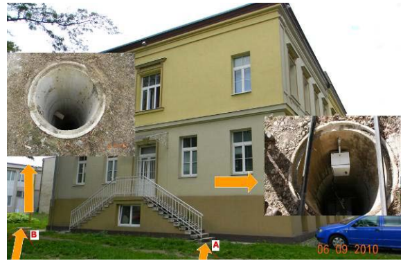
Fig. 4 location of infiltration shafts near building PK6
