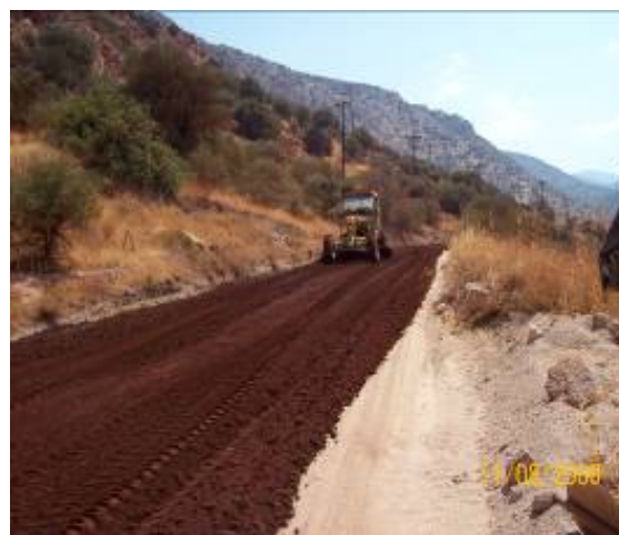
Fig. 4: Spreading the material (2009)
