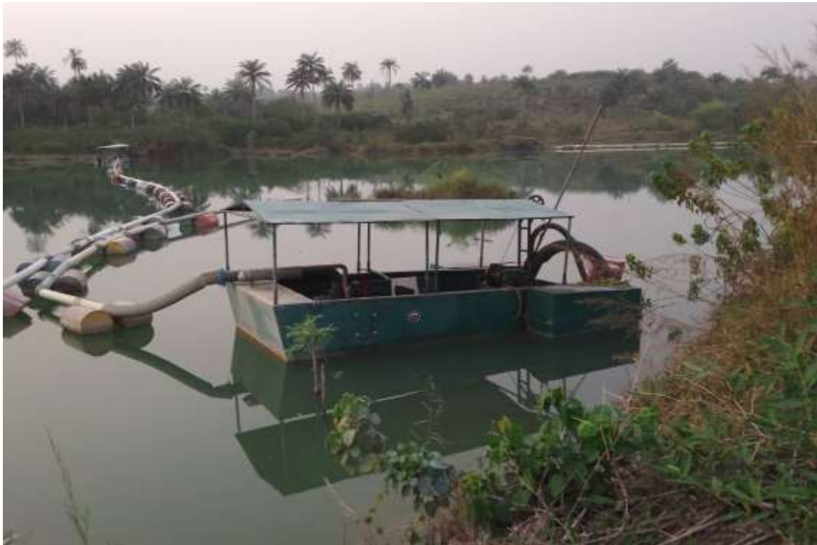
Figure 1: Rolls Royce dredging machine connected to a suction pipe
