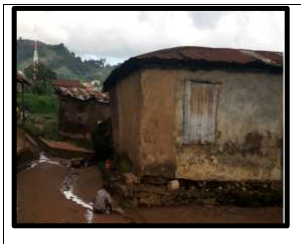
Fig. 4: A Typical flooded building at Irona Street, Ado-Ekiti
