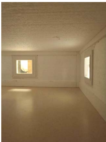
Figure 9: Polystyrene wall and ceiling viewed from inside.
