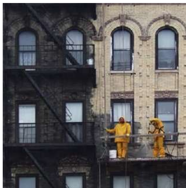
Fig. 3: Colour contrast of building surfaces affected by CO [4]
