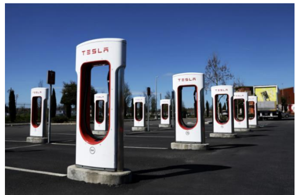
Fig. 1: Tesla charging stations. The station with plugged-in EVs can be exploited as a clustered energy storage to support the power grid Source: [14].
