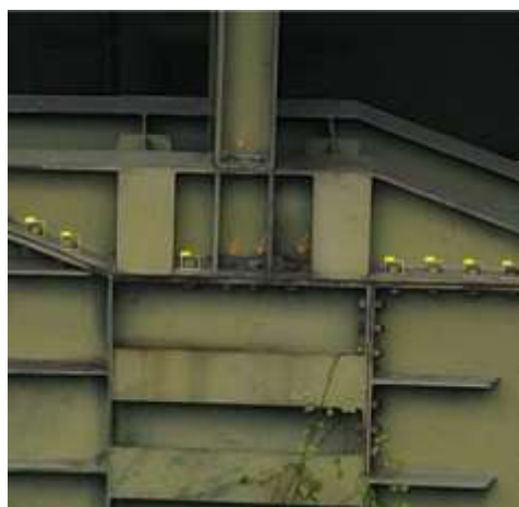
Fig. 7: Zoom on an area with processing problems - red arrows indicate bolts not recognised by the processing system.
