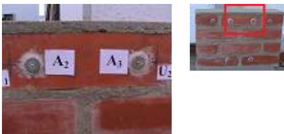
Fig. 16: Detail of a zone of interface between mortar joints and bricks (vertical and bed joint) in face A of the Specimen M1 at the end of 3 rd Phase of the test
