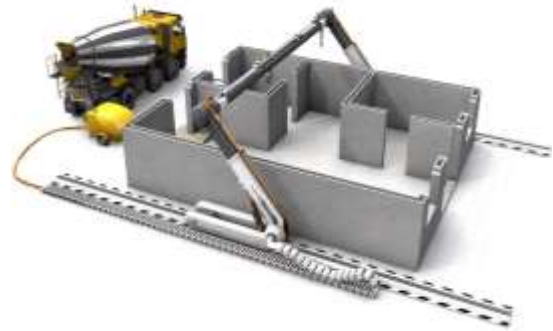
a) a printer working directly on the construction site
