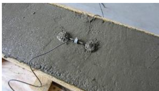
Fig. 5 – Detail on installation of external string strain gauge.
