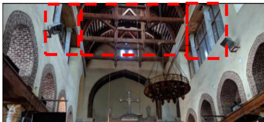
Figure 3: Roof structure, windows and arches of St. Barbara church. Source: [33]
